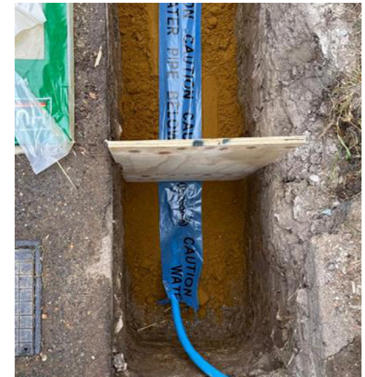
Pipe bedded down with sand
