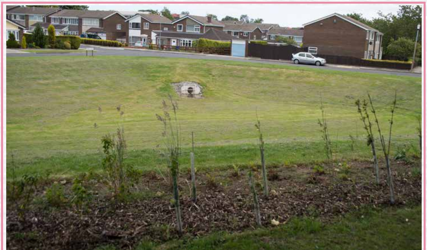
Figure 3: Detention Basin, Megstone Avenue, Cramlington
