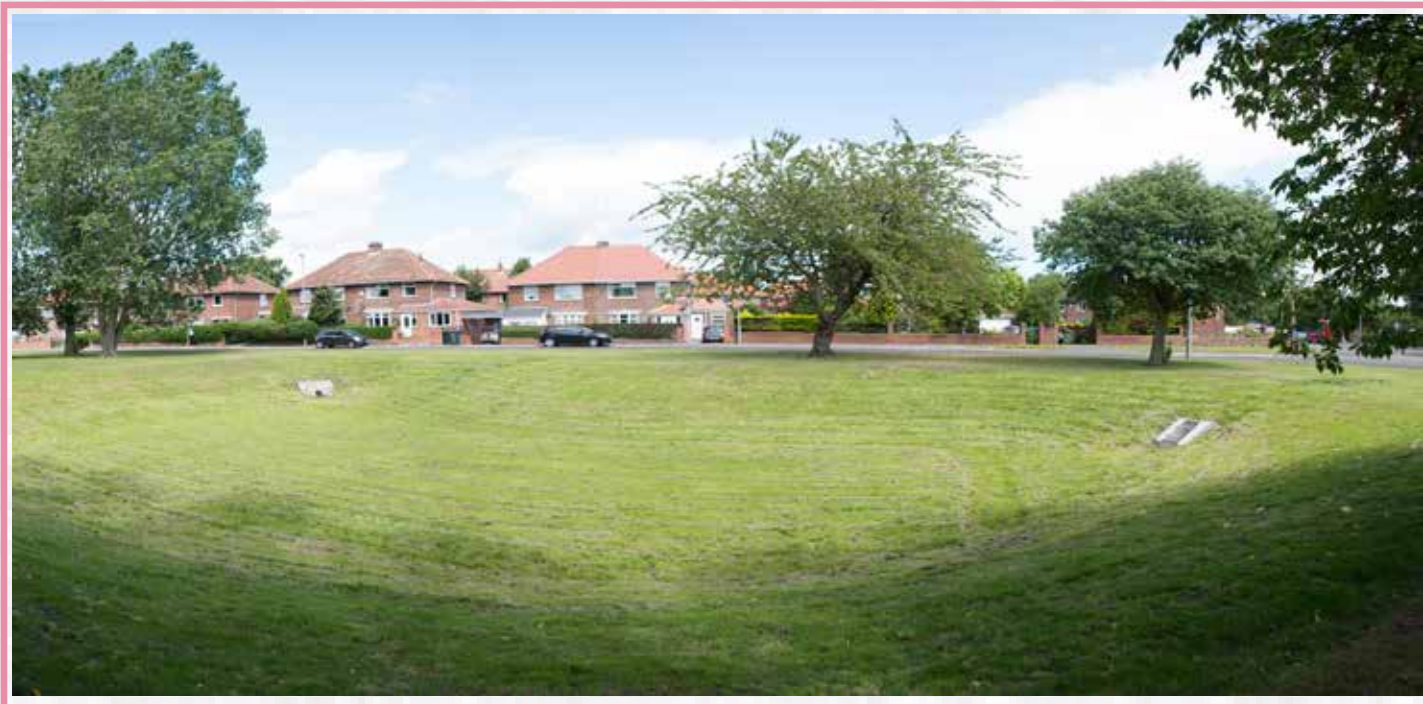
Figure 3: Completed detention basin.
