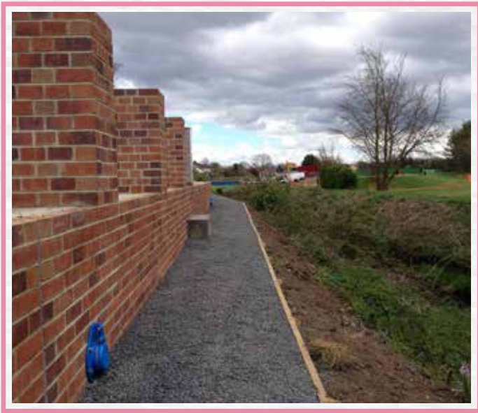
Flood defence wall and existing Ouseburn
