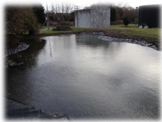
Refurbishment of an existing pond at Newton Aycliffe treatment works
