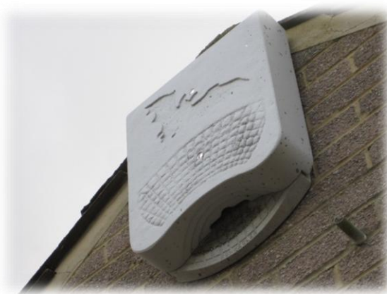
Installation of a summer and winter bat roost at a County Durham sewage treatment works
