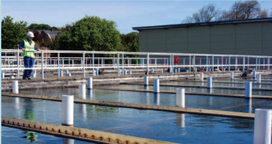
Horsley water treatment works in Newcastle upon Tyne.
